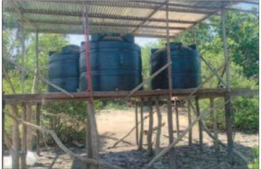
Three water tanks, including one containing petrol, seized by Marine.
