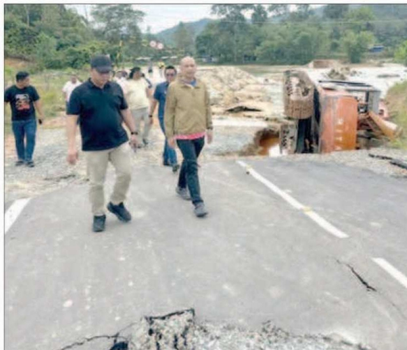
Armizan (middle) visiting the collapsed the low-level crossing at Kg Kaiduan.
